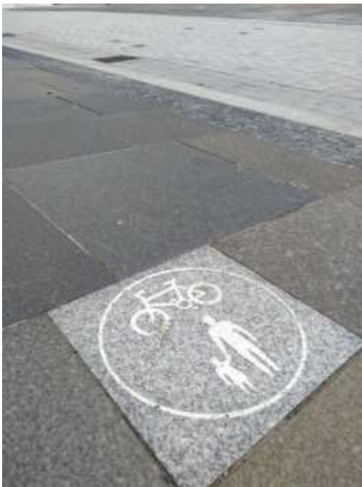
L: current setts on Broad St of TSRGD Diagram 956. ACC may consider replacing these with symbols depicting people, if shared footway is removed.
